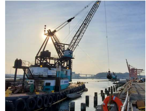
USACE Sargent Beach Jetty and Beach Renourishment Project
