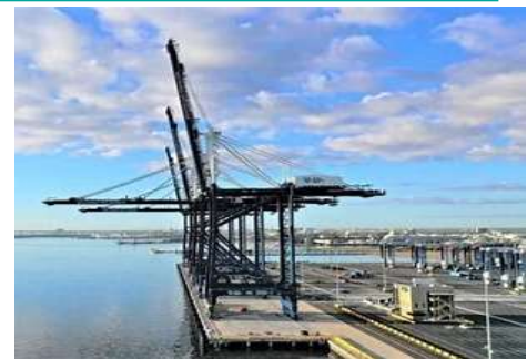
Terminal Wharf Expansion
