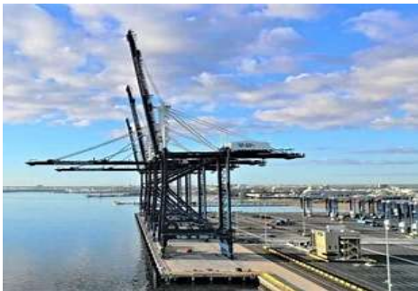
Terminal Wharf Expansion
