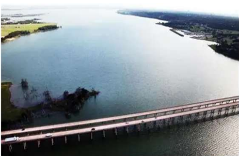
Bridge Replacement Contract in Texas
